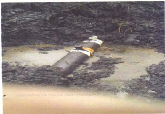
REPAIR WORK DONE BY NAOC REPAIR TEAM
